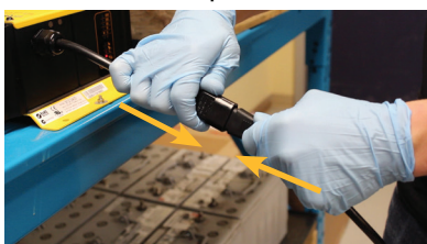
Figure 3: Reconnect AC power to the charger.
