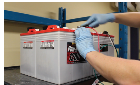
Figure 8: Reattach the positive lead to the positive terminal after disconnecting AC power.
